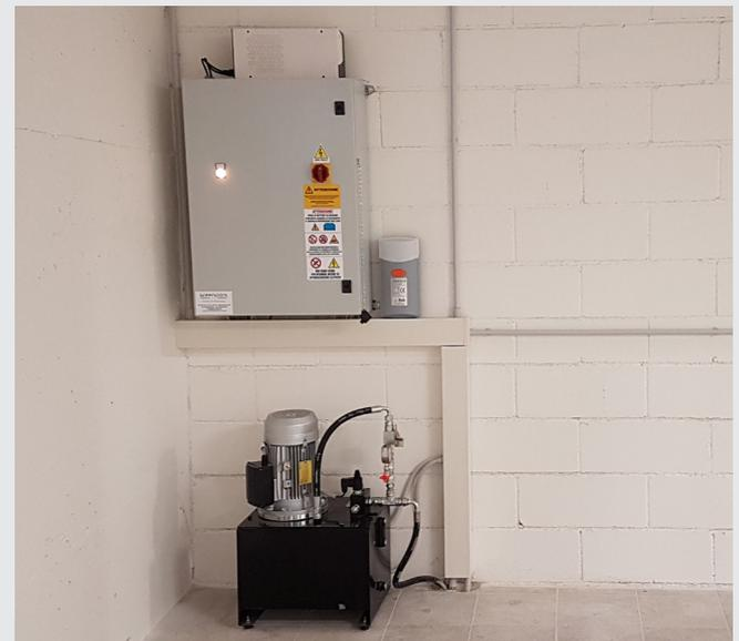
QUADRO MACCHINA E CENTRALE IDRAULICA
